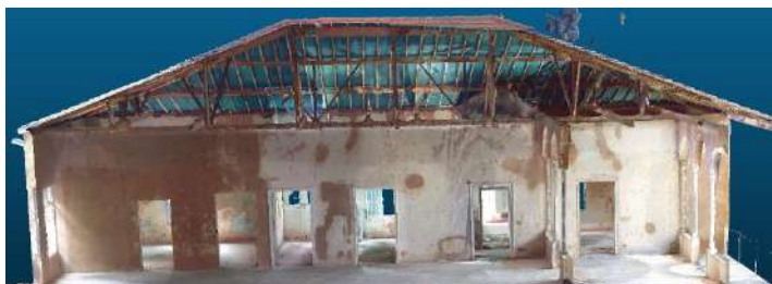
3D Model and 3D sections by Laser scanning
