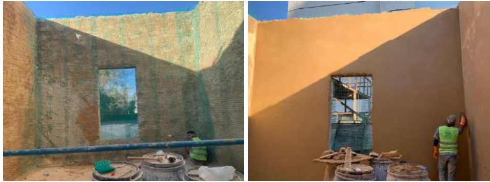
Structural Plastering
