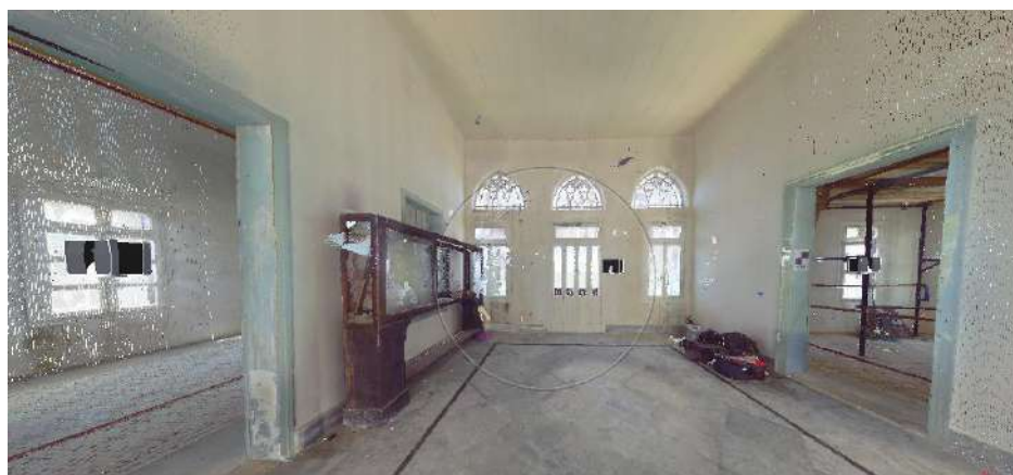
Laser scanning point cloud output
