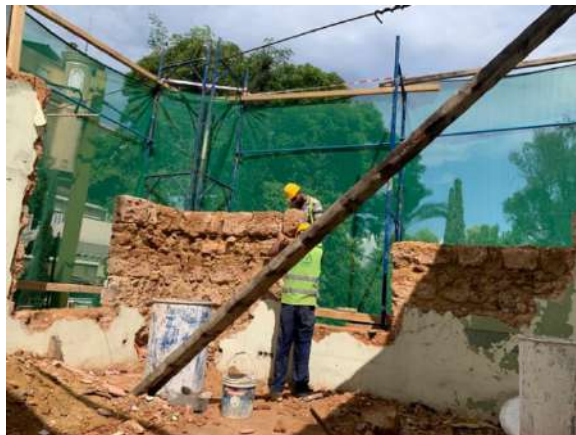
Dismantling and remounting walls
