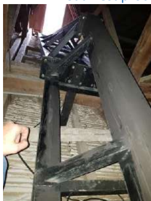
Steel truss supporting the Luster
