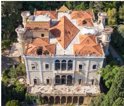
Sursok palace Beirut damaged by the Beirut blast 2020 – North Façade Out of Plane deformation 25cm
