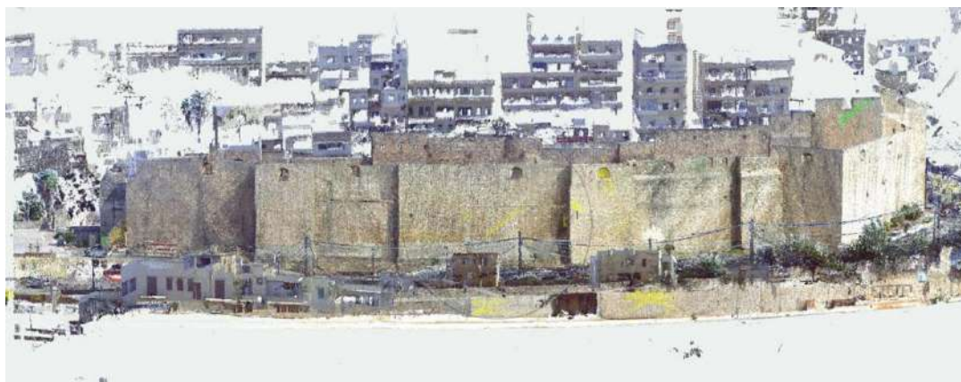
Laser scanning point cloud output
