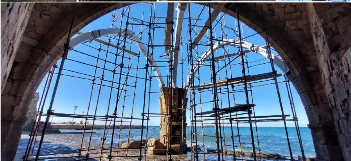
Consolidation of the demolished part of the vault
