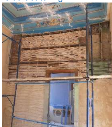
Cracks stitching
