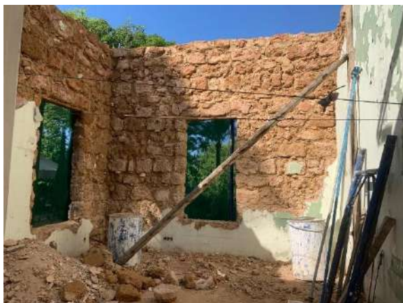
Dismantling and remounting walls
