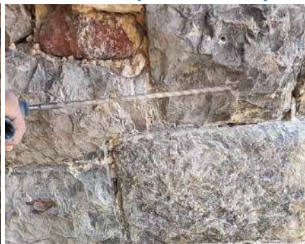
Strengthening a vault edge
