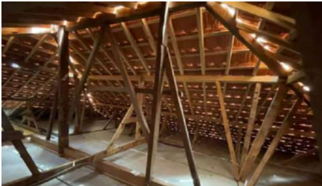
Wooden attic repair
