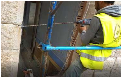
Threaded rods for corners reinforcement
