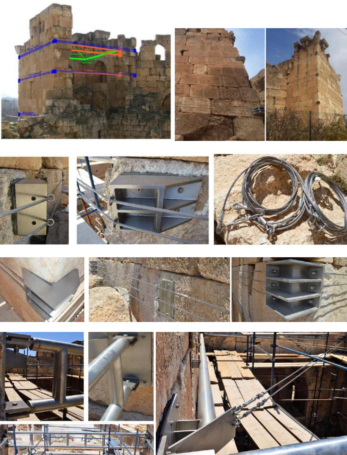
ARAB TOWER – BAALBEK: CONCEPT OF THE CONSOLIDATION SYSTEM AND DETAILS
