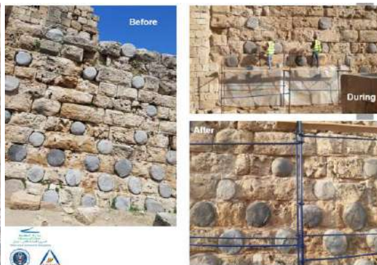
Walls of the main entrance
