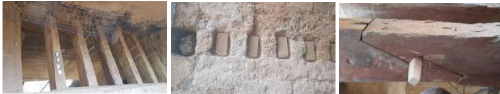
Wooden beam repair
