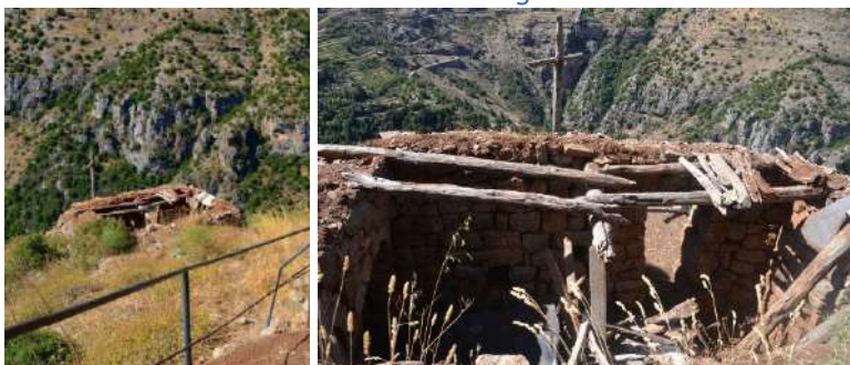
St James Church before restoration
