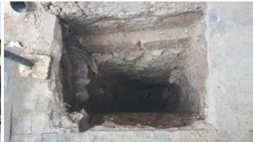
Foundation inspection pit
