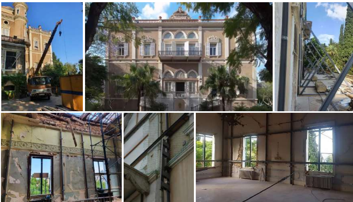
Sursok palace Beirut damaged by the Beirut blast 2020 – North Façade Out of Plane deformation 25cm
