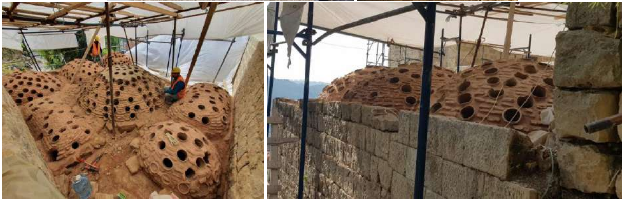
Restoration of Hammam historic domes
