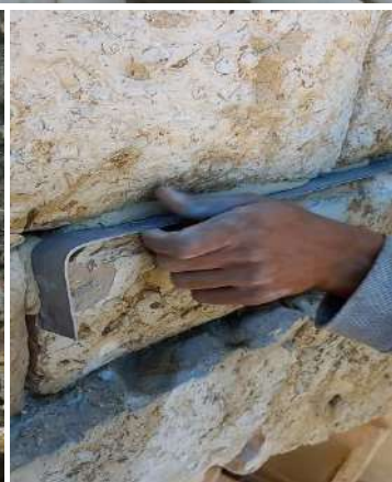
Cracks stitching
