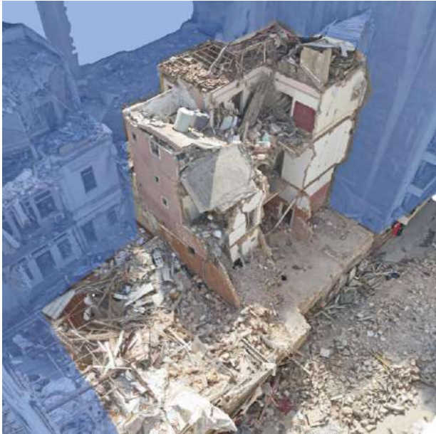
Scale of destruction of the building following the blast - Collapsed part of Rmeil 733
