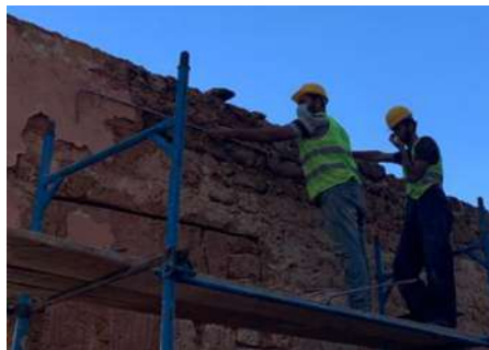
Stitching of structural cracks
