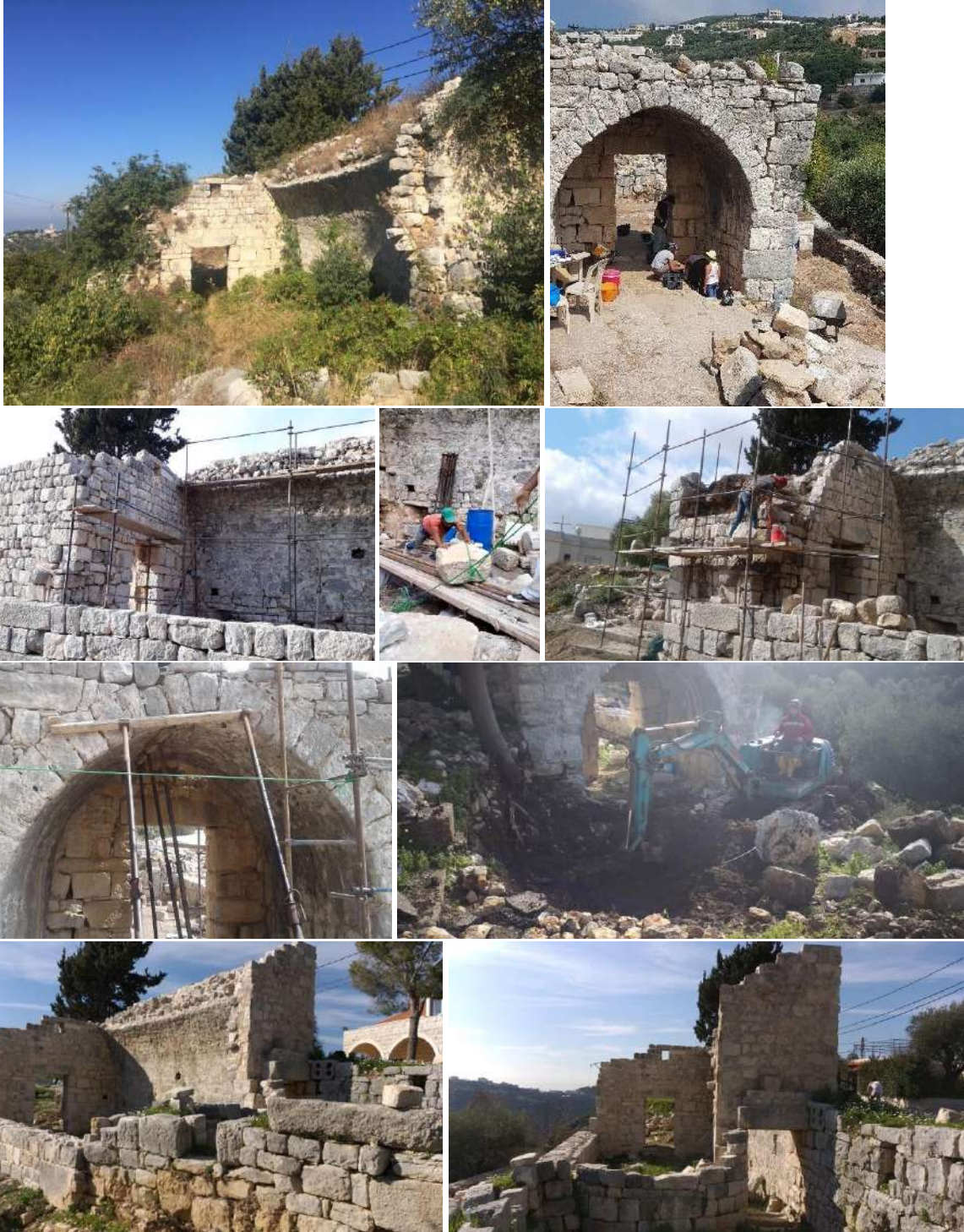
St Nicholas Behdaydet – During execution
