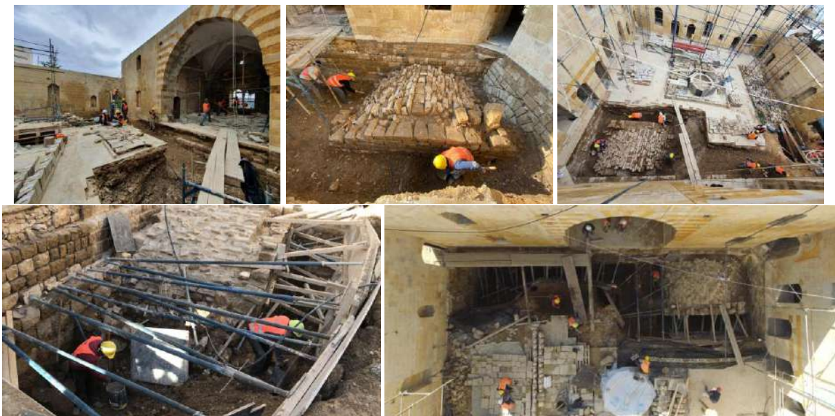
Excavation of the main court
