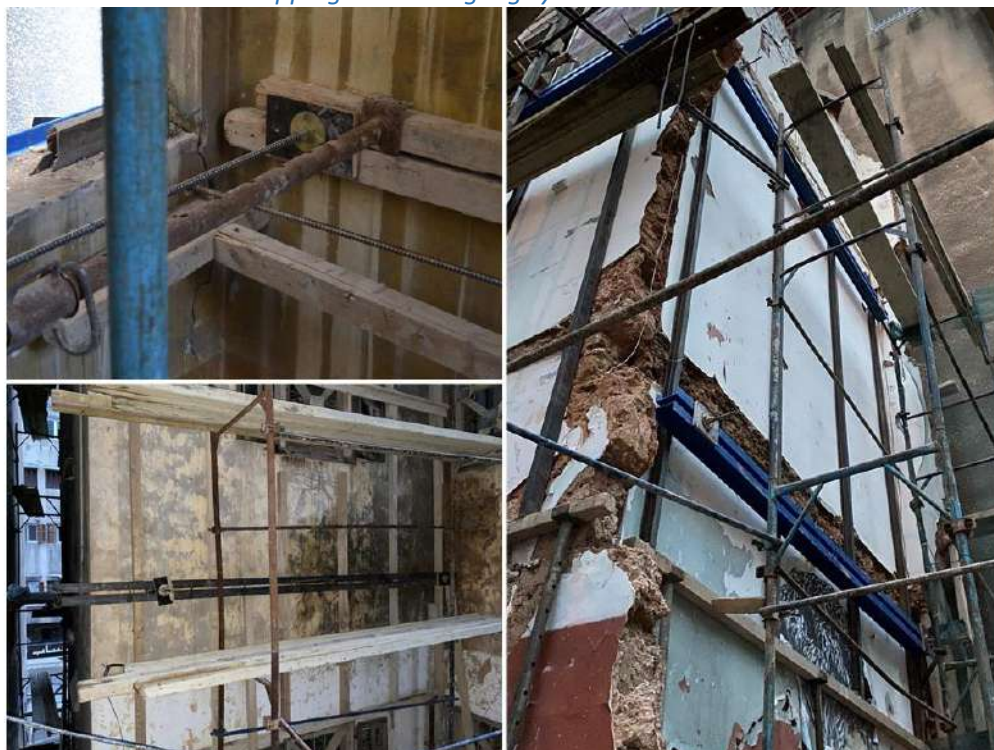
Tie rods strengthening systems
