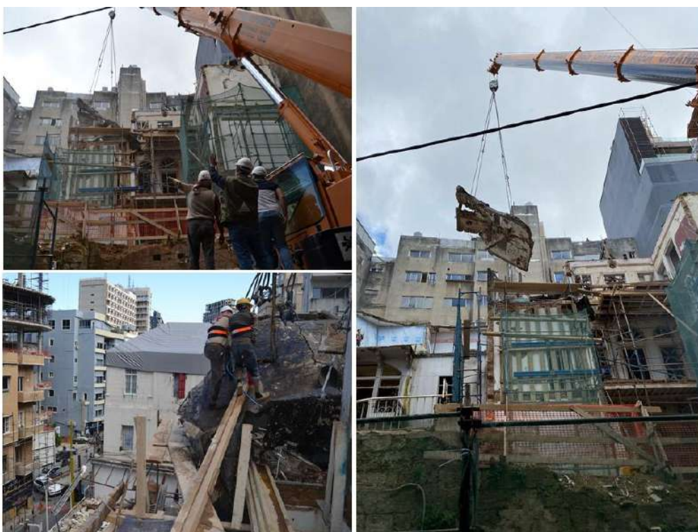
Removal of the collapsed concrete slab
