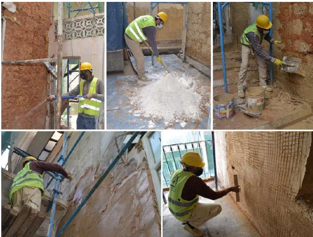
Re-plastering process
