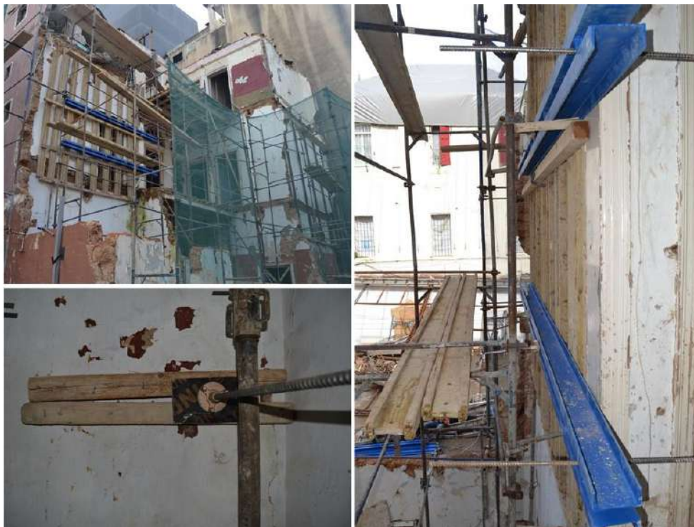
Tie rods strengthening systems
