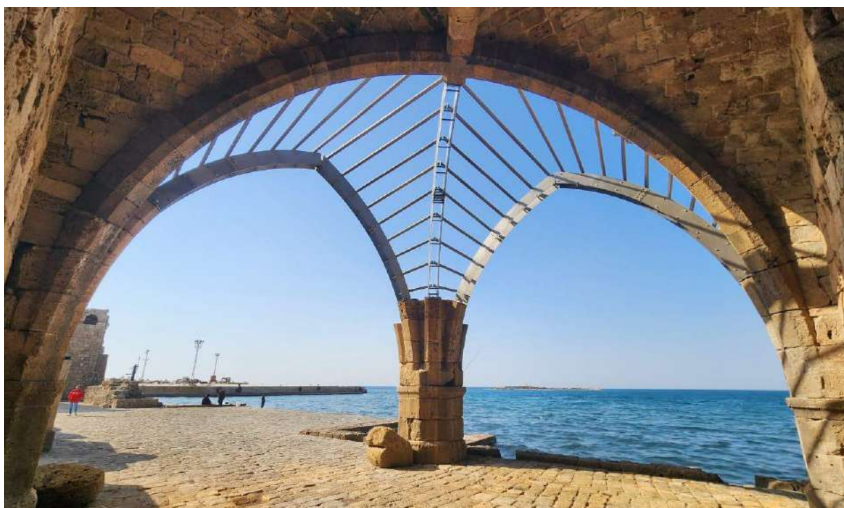
Final state of the consolidated vault
