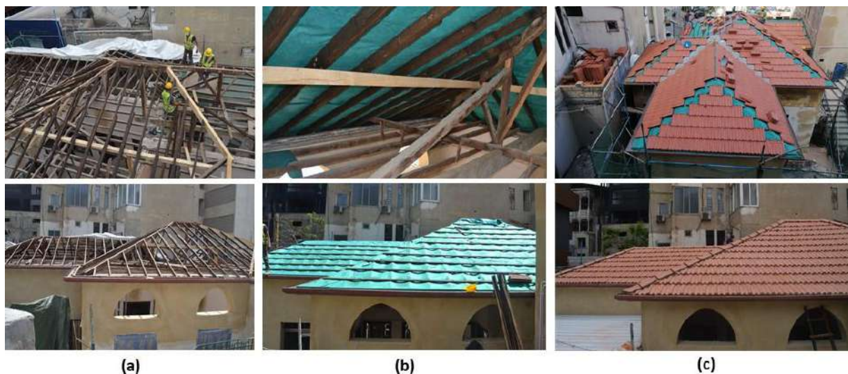
Attic consolidation, (a) replacement of damaged timber elements, (b) Mesh installation to avoid water infiltration, (c) Red tiles installation
