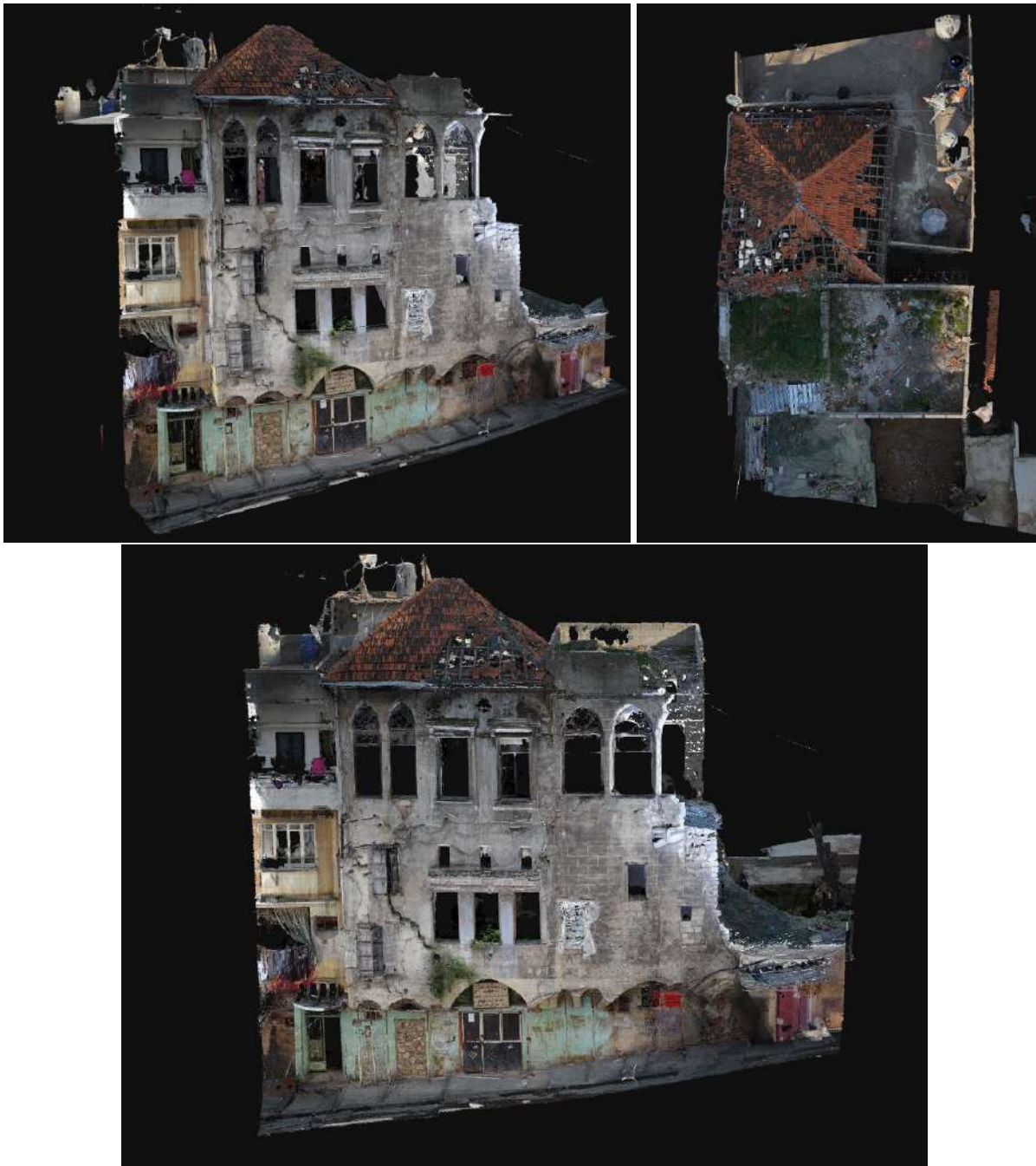
3D Model by combination of laser scanning and photogrammetry
