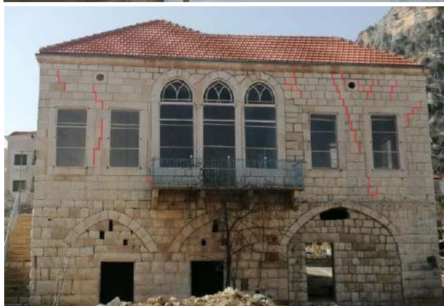
Structural cracks
